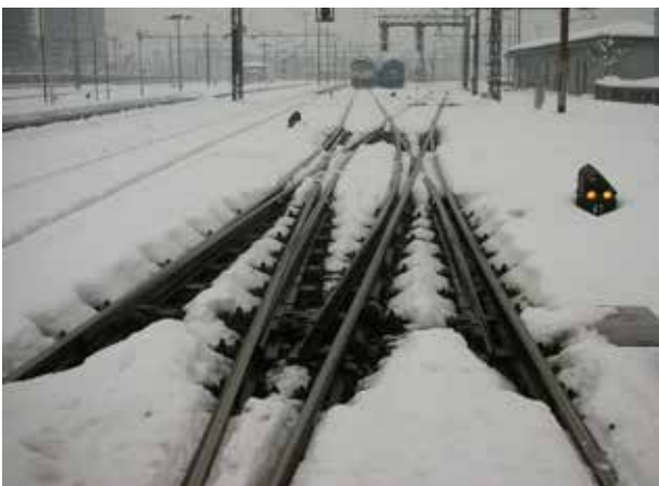
Typical Heated Points Systems - Milan, Italy.
